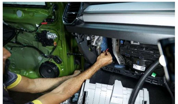
STEP 52 :- AFTER ROUTING THROUGH THE HOLE, PULL ALL THE EXCESS CABLE GENTLY
